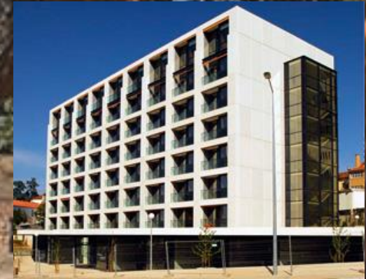
Studio Residence - Coimbra
