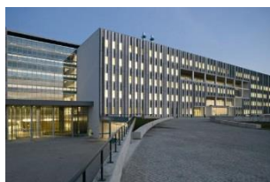
Novo Hospital de Braga
