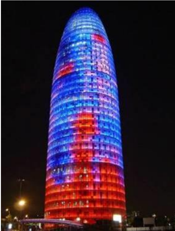
Torre Agbar parking, Barcelona 20.000 m 2 C-FLOOR
