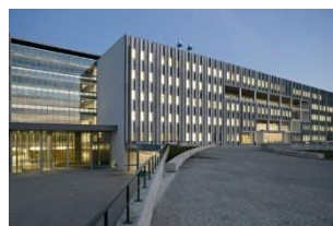
Novo Hospital de Braga
