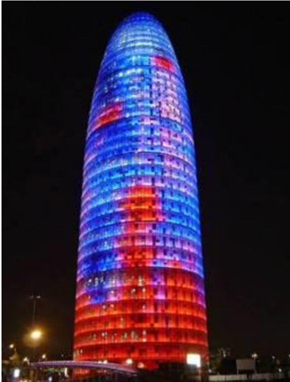
Torre Agbar parking, Barcelona 20.000 m 2 C-FLOOR
