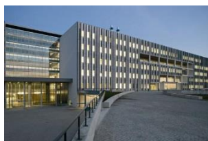
Novo Hospital de Braga
