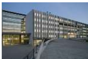
Novo Hospital de Braga
