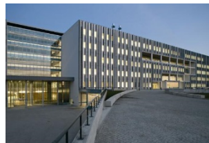
Novo Hospital de Braga
