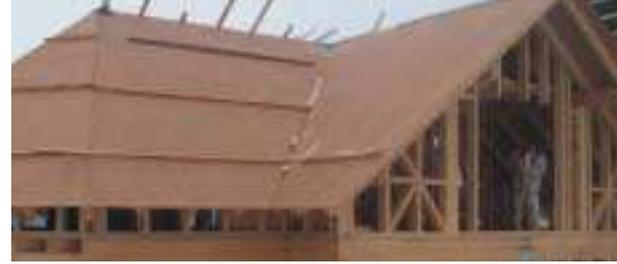
The AGEPAN® DWD protect used as a structural board in the wall.
