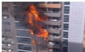
Torre Saif Belhasa, Dubai, 2012
